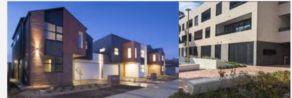
FIGURE 9. EXAMPLE OF DIVERSE HOUSING TYPES (TOWNHOUSES AND LOW-RISE APARTMENTS)
